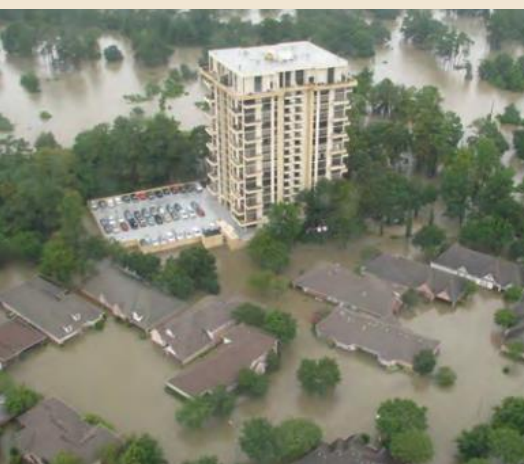
Flooding of Cypress Creek near Champions Forest Drive. Hurricane Harvey. Photo Credit: HCFCD.
